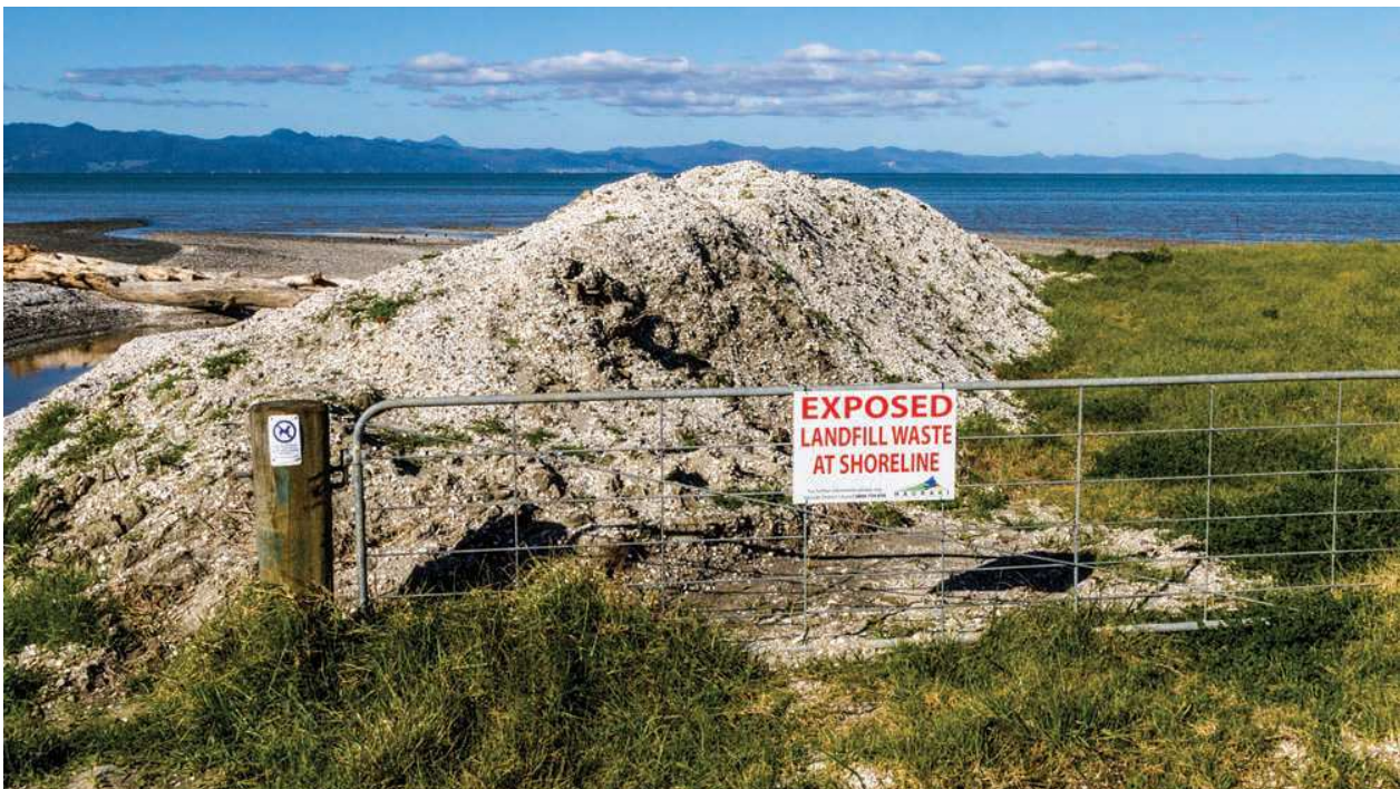
The NZCPS addresses the restoration of natural character including the decommissioning or restoring of historic landfills such as this one on the Kaiua coast, Firth of Thames (Raewyn Peart)
