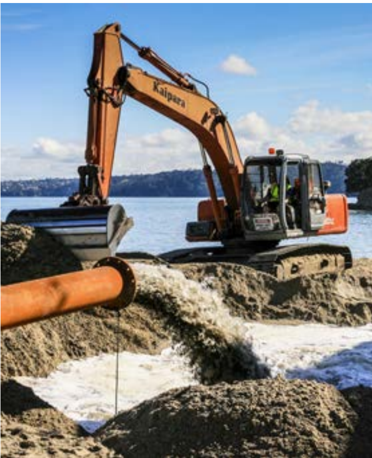
Beach replenishment, Point Chevalier, Auckland
