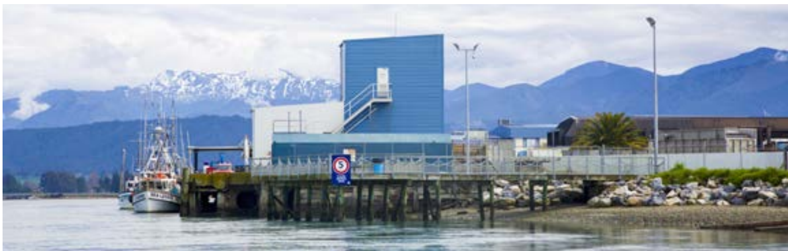
Seafood processing plant, Motueka
