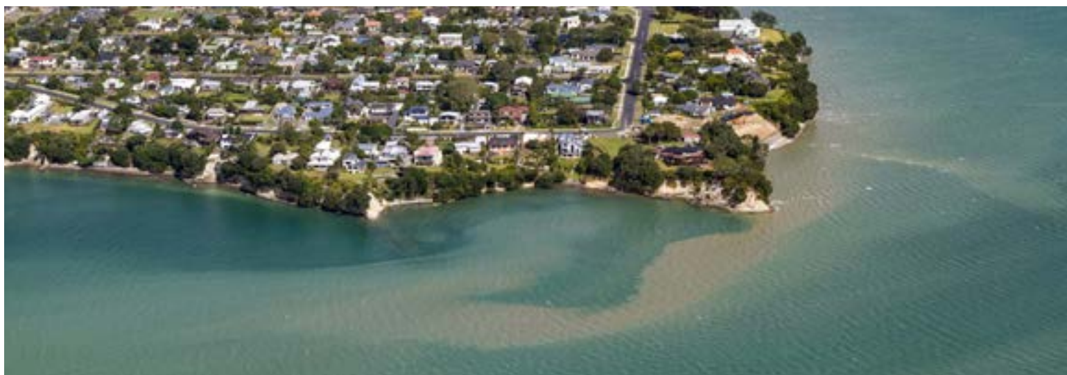
Sediment-generating earthworks, Beachlands, Auckland
