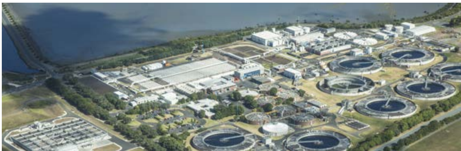
Mangere wastewater treatment works
