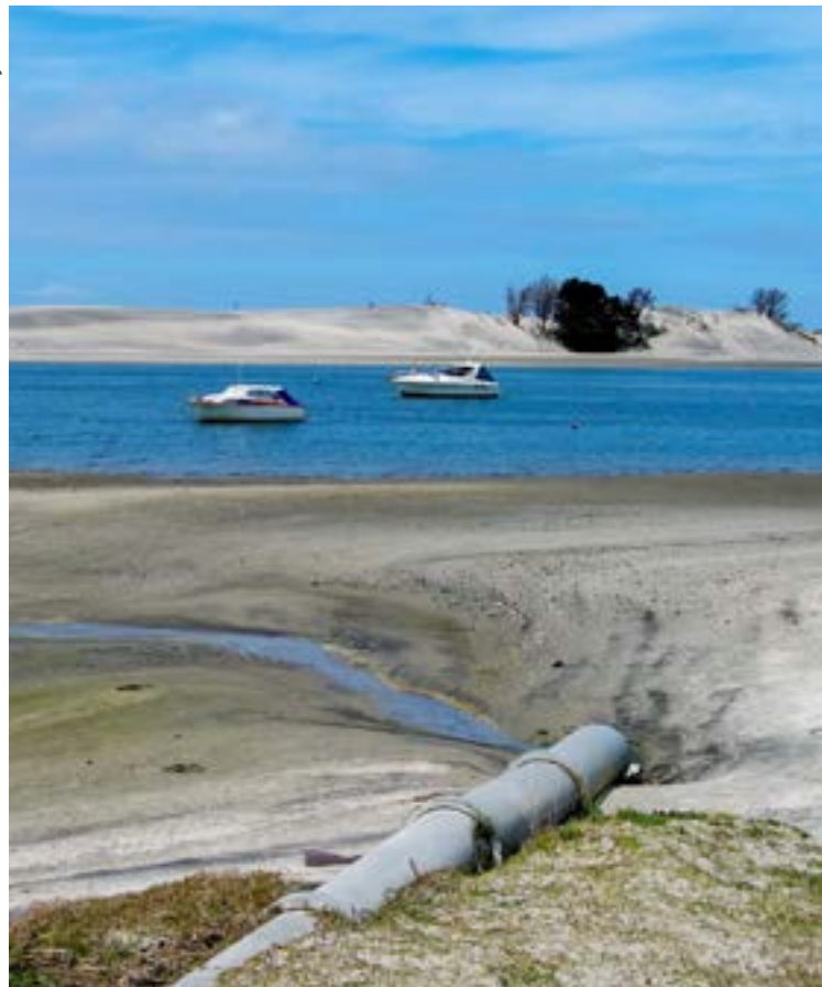
Stormwater outfall, Mangawhai
