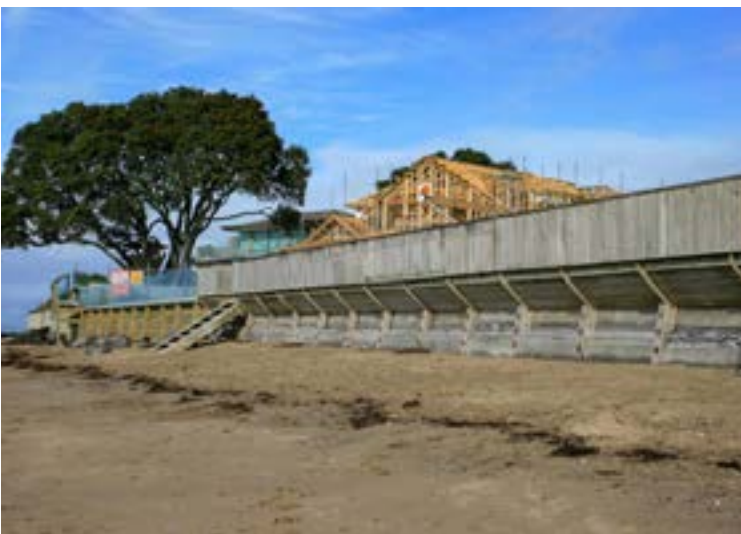
Seawall, Milford, Auckland
