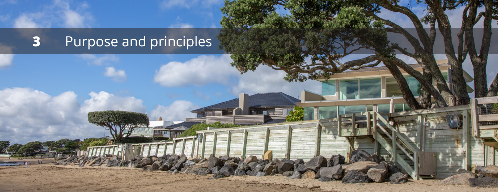
High value homes protected by seawalls at Milford Beach, Auckland
