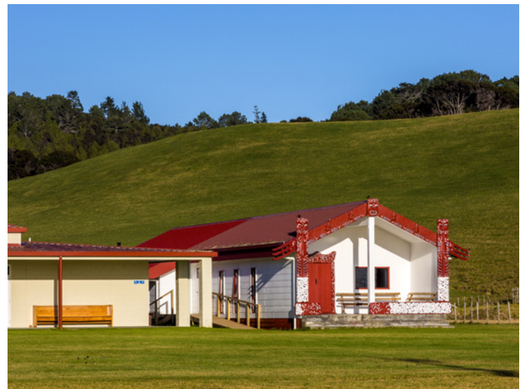
Umupuia Marae which is subject to flooding
