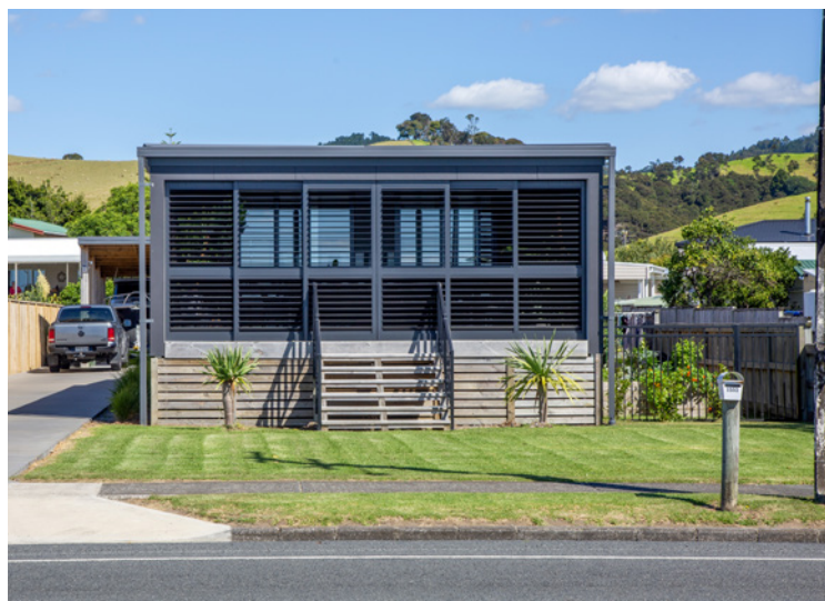
A house located in a part of Kawakawa Bay which has previously flooded has been raised onto higher foundations as an adaptation measure
