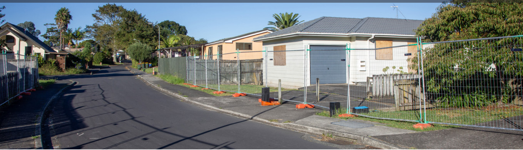
Houses at Clover Drive, Henderson, Auckland vacated due to the Auckland Anniversary Floods
