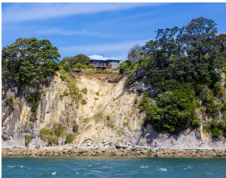
Coastal cliff erosion at Ferry Landing, Whitianga
