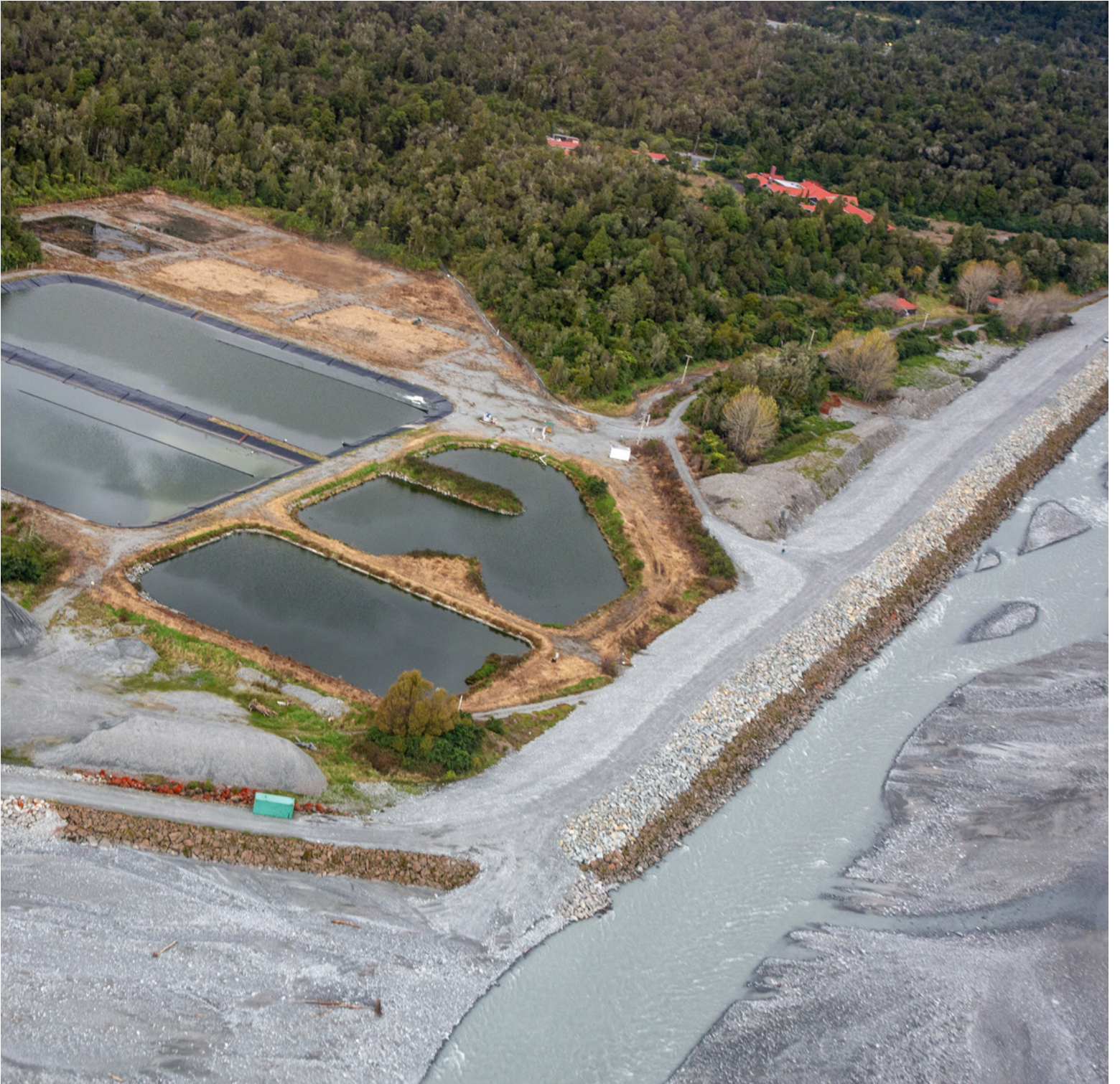
Stopbank on the Waiho River protecting Franz Josef wastewater treatment plant
