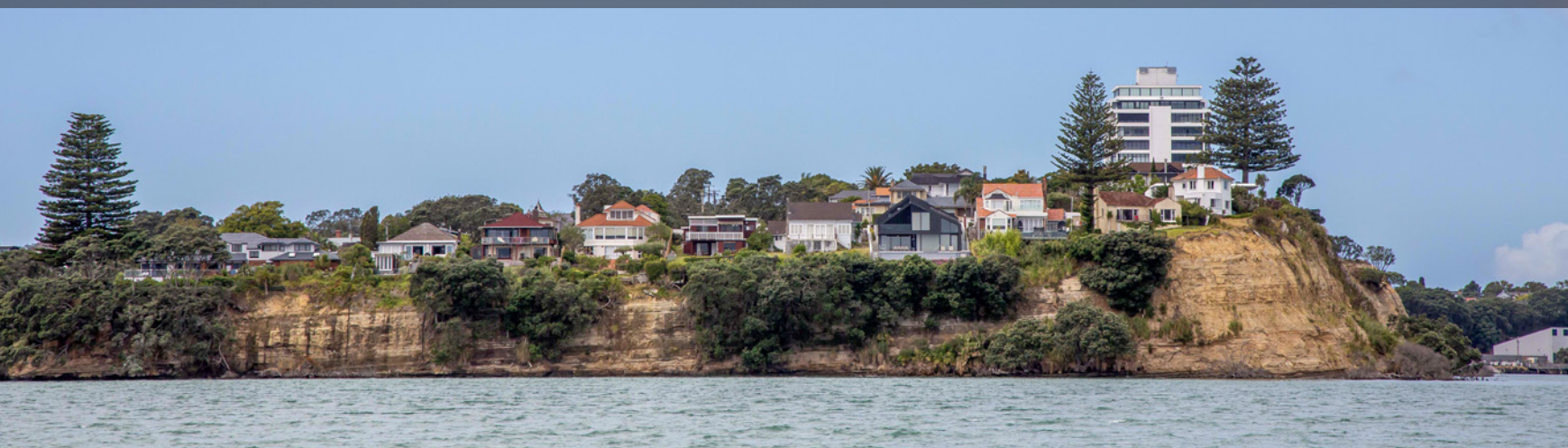
Eroding coastal cliffs, Stanley Point, Auckland
