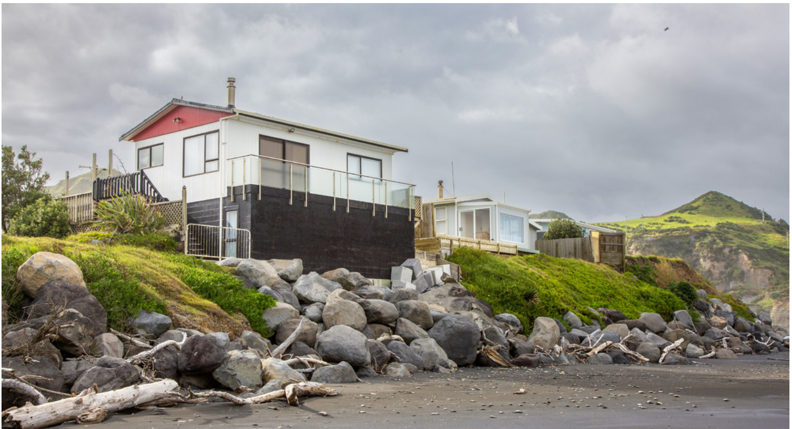
Coastal erosion at Mokau
