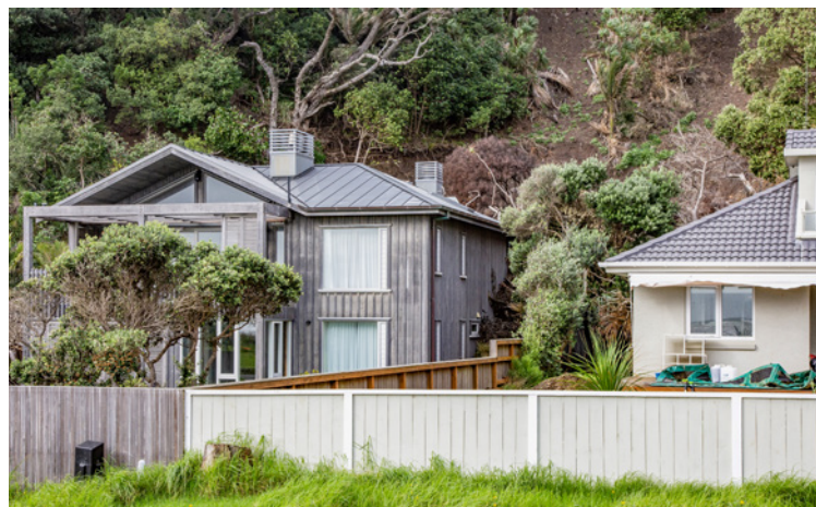
Vacated houses in South Piha due to slip damage
