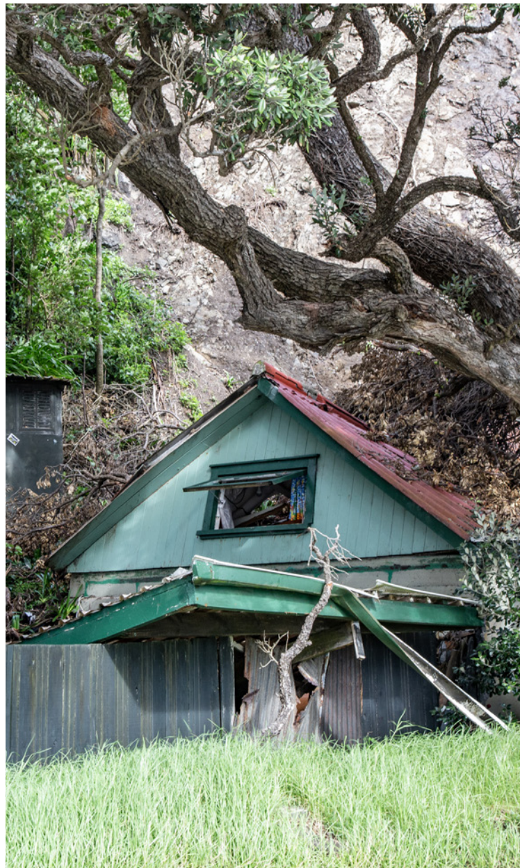
Slip-damaged house at Piha, Auckland
