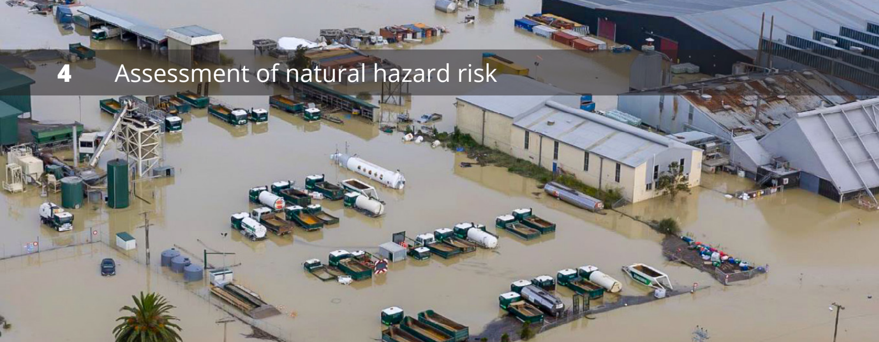
Flooded contractor's yard, Hawkes Bay (Waka Kotahi)
