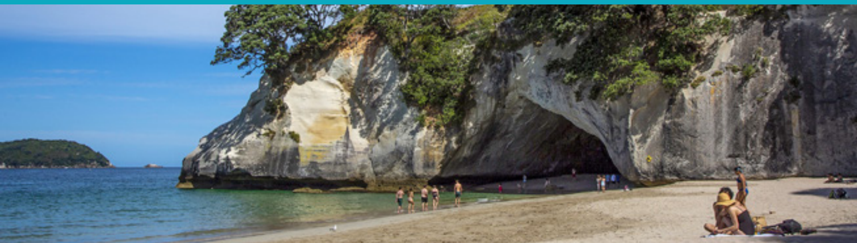
Cathedral Cove, Hahei. Damage from Cyclone Gabrielle led to closure of the track to the Cove and DOC is coming under strong pressure to repair and reopen it due to the impact of closure on tourism revenues
